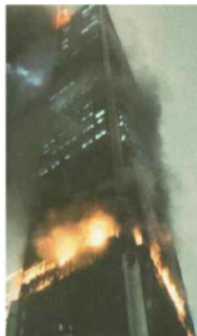
LA Interstate Bank Fire
